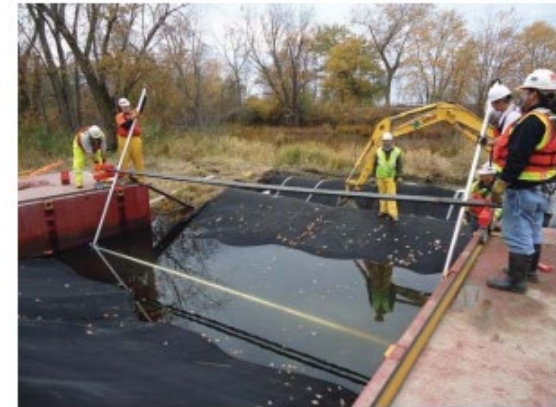
Placement of geocomposite
