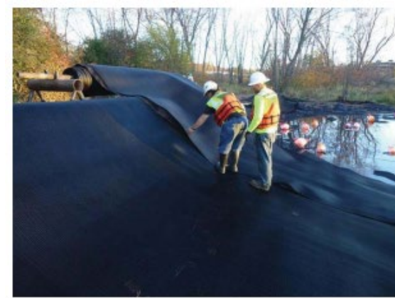
Seaming geocomposite panels
