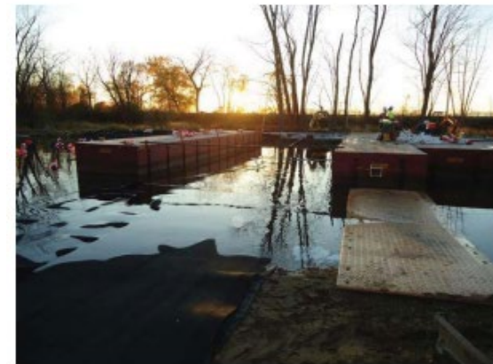
Photograph of barge configuration of geocomposite placement
